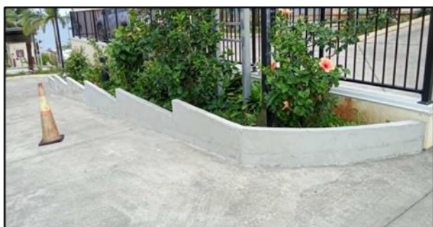
Figure 5: Newly raised concrete flower bed, awaiting top soil placement, painting and introducing of new flowers.
