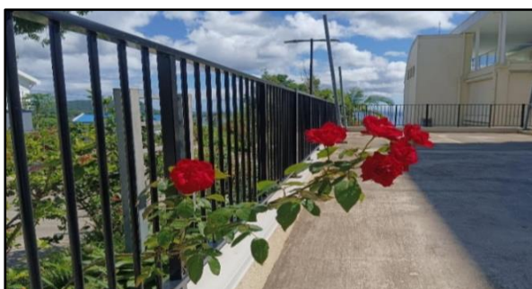
Figure 2: Parking lot iron fencing.
