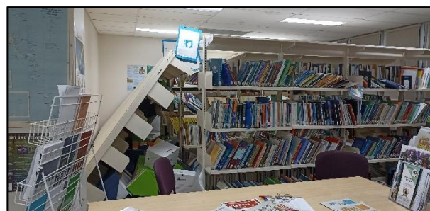
Figure 13: Damage in the library by the devastated earthquake in the last quarter of 2024.
