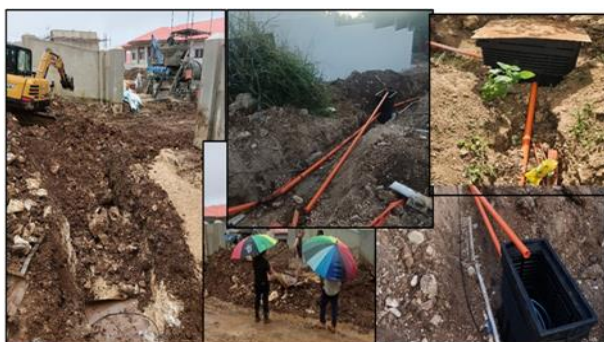
Figure 3: Excavation by CGGC and connectivity re-route and completion work by PACNET at Presidential Palace Main Entry.
