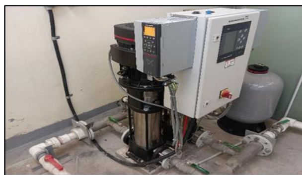
Figure 1: New booster pump – replacement job by South Pacific Electrics.
